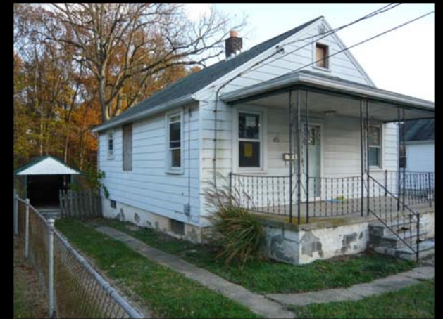
Original Single Story House
